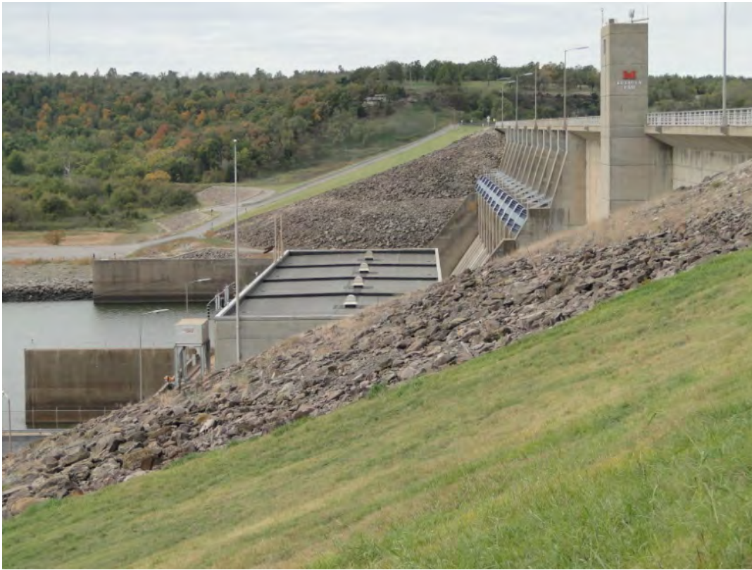
Figure 3.10-3. Prohibited Access Area at Eufaula Dam
