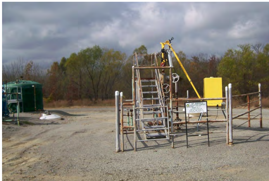
Figure 3.4-2. Natural Gas Well at Eufaula Lake
