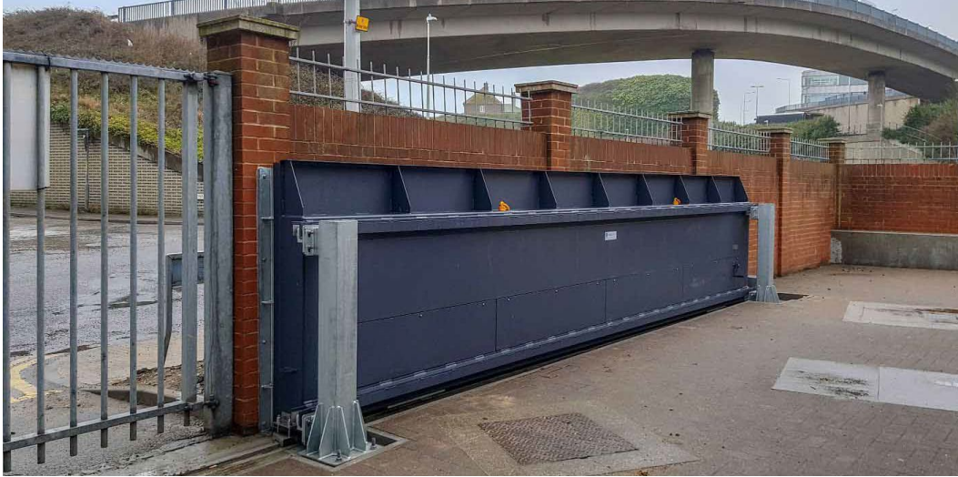
Figure B-48: Typical Roller Gate
