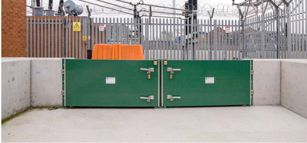
Figure B-47: Typical Swing Flood Gate
