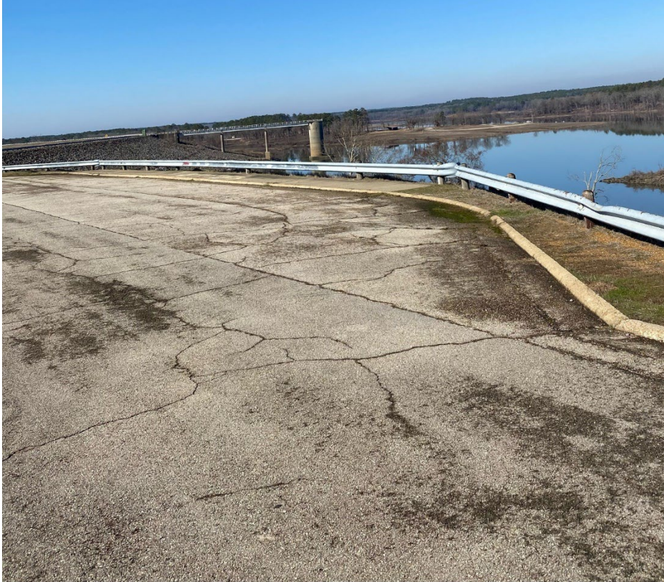
Photo 5.1 Overlook area (Source: USACE)
