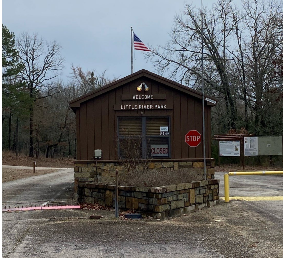
Photo 5.4 Gate house at Little River Park (Source: USACE)
