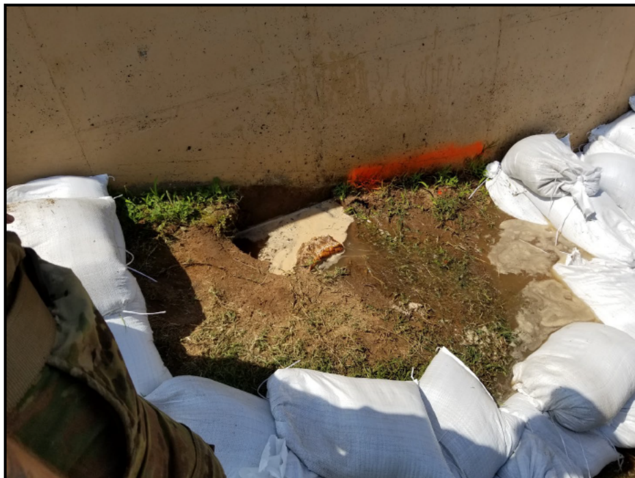
Figure A-7: Erosion at Charles Page Floodway Structure
