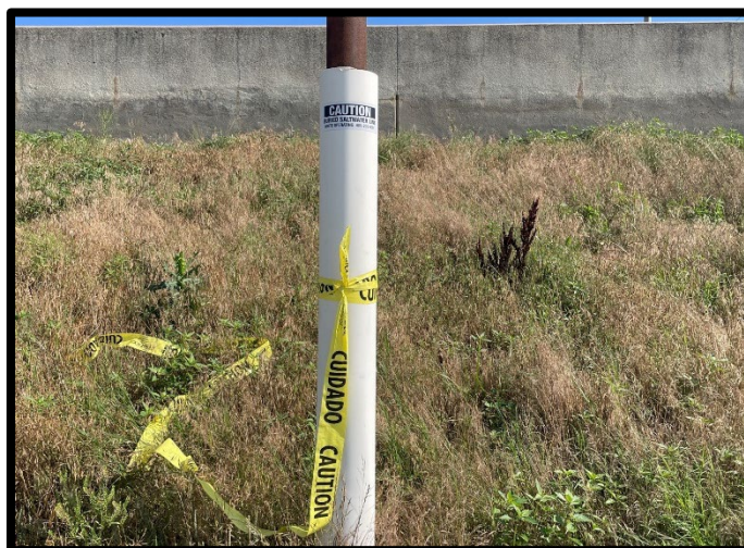
Photo 3: Buried Salt Water Line Marker
