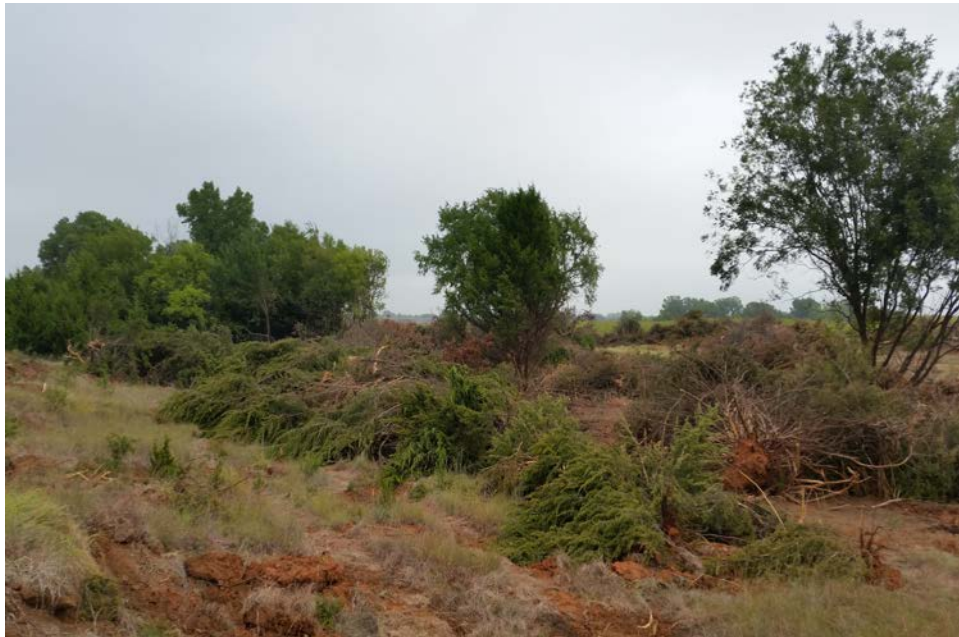
Photo 2. Tree removal in the area of the water storage tower location, view to the north.
