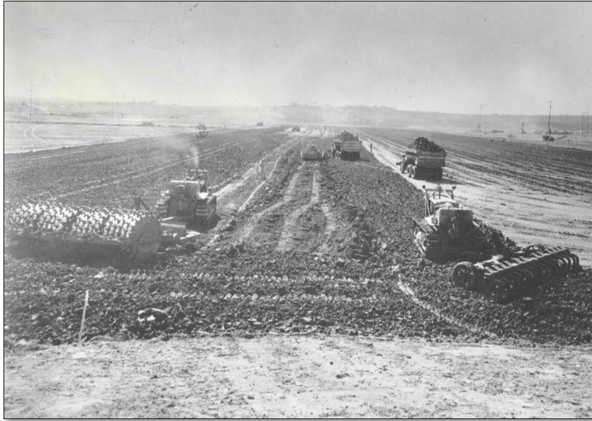
Figure 9. October 17, 1940, photograph of the construction process of placing, moistening, and rolling the materials that make up the interior of the dam embankment.
