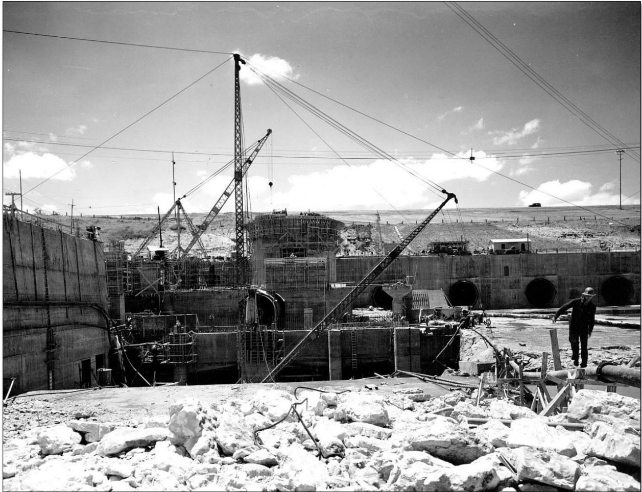
Figure 21. June 11, 1943, photograph of the progress on construction of draft tube forms for powerhouse.
