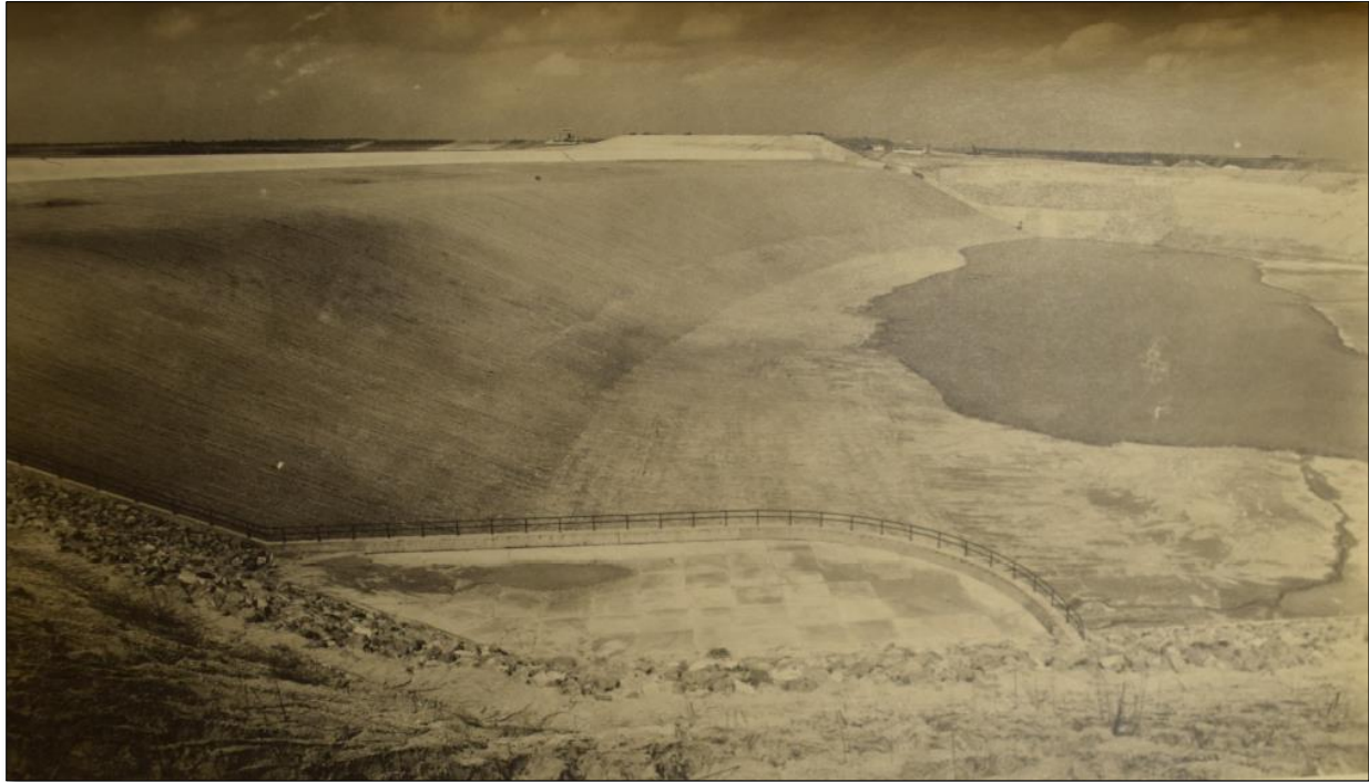
Figure 17. March 26, 1944, photograph of the completed spillway and stilling basin.
