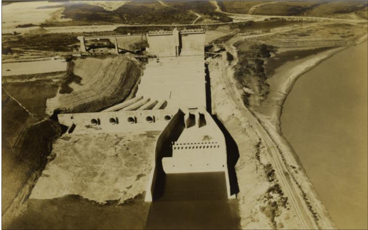
Figure 22. October 10, 1941, photograph of outlet works (center), stilling basin (foreground), and intake structure (background) as construction neared completion. Ultimately, the powerhouse was constructed at the left side of the foreground (in front of the conduit openings visible in the photo) and the dam embankment filled in over the top of the flat concrete area in the center of the photo.
