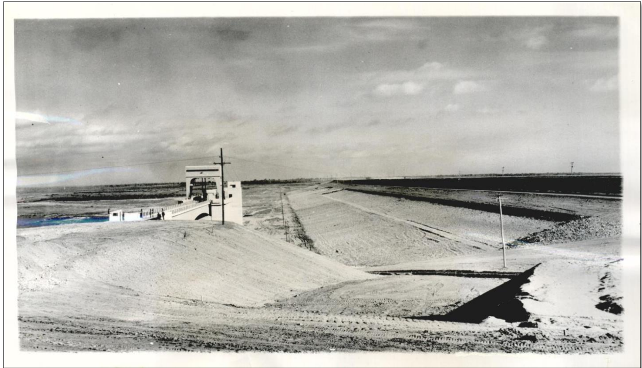
Figure 11. November 26, 1943, photograph of the reservoir side of dam embankment (at right side of photo) before placement of the limestone riprap.
