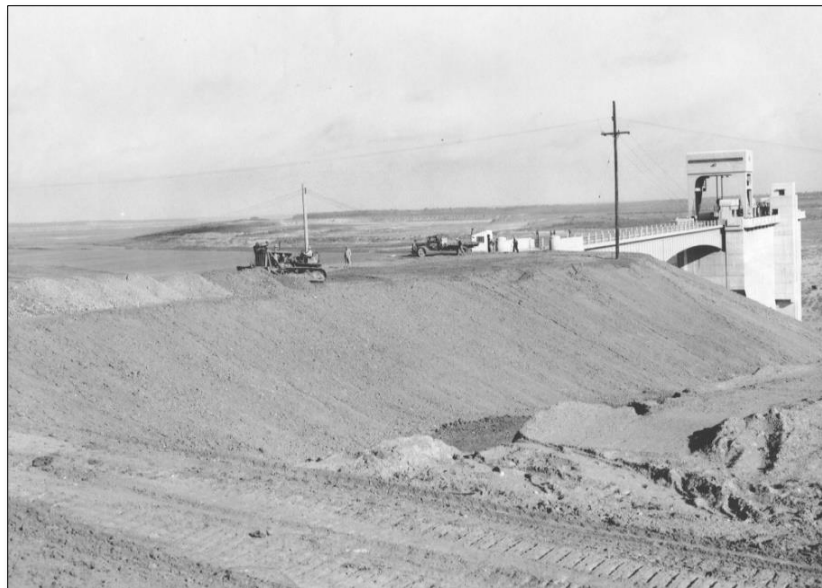
Figure 20. October 19, 1943, photograph of the intake structure that directs water into the outlet works' eight conduits. It is located upstream from the dam embankment.
