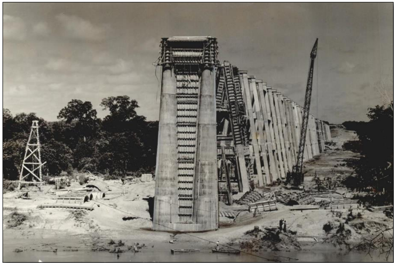
Figure 33. July 23, 1943, photograph of the substructure of the new bridge to carry a relocated railroad over the Washita arm of the reservoir.
