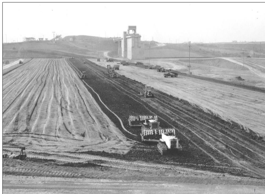
Figure 10. February 1, 1942, photograph of crews placing and rolling the impervious fill materials for the dam embankment.
