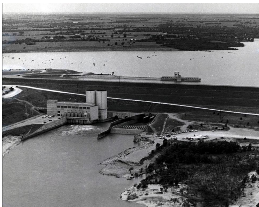
Figure 28. Ca. 1950 overview photo of Denison Dam, intake structure, powerhouse, and outlet works.
