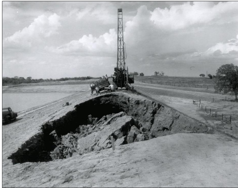
Figure 16. May 28, 1957, photograph of a Denison Core Barrel being used to take samples at flood prevention dam no. 7 on Owl Creek near Purcell, Oklahoma, to determine the cause of the failure shown in the photo.
