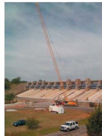
Canton Lake, Oklahoma, Dam Safety Project
