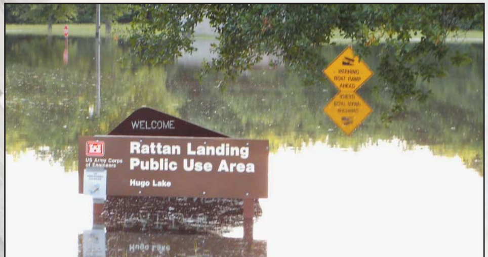
High water at Hugo Lake, Oklahoma, reflects the signs at the Rattan Landing Public Use Area. The high water resulted in closed campgrounds and facilities. Nearly all of Tulsa District's 33 lakes were impacted by the wide-spread storms of June and July.
