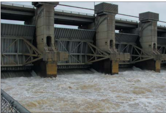
Copan Lake water releases through the spillway.
