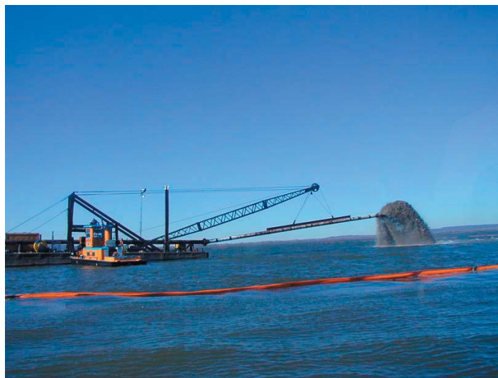
Dredging the McClellan-Kerr Arkansas River Navigation System is an ongoing maintenance need to keep the channel open. The ongoing deepening project will allow shippers to increase the loads hauled. The greater capacity of the channel the greater system efficiency.
