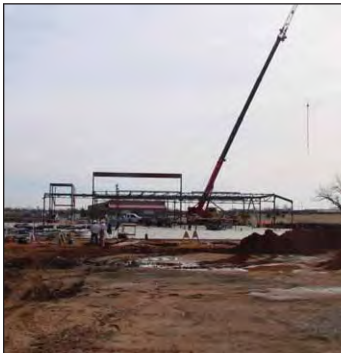
Air Defense Artillery School dining facility under construction at Fort Sill.
