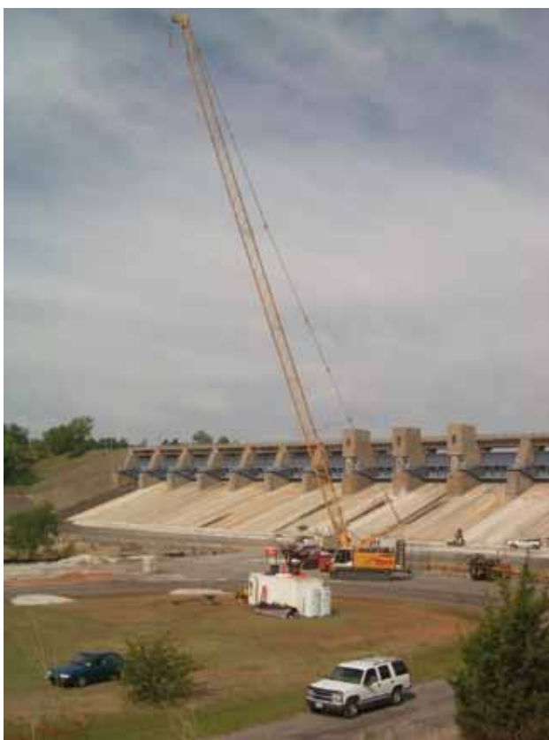
Canton Lake, Okla., Dam Safety Project
