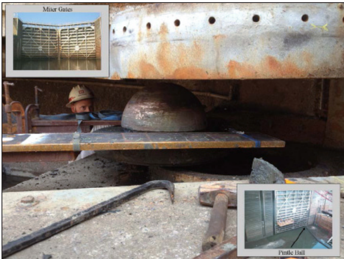
Shane Roe, team lead for Tulsa District’s maintenance crew on this project, checks out a pintle ball at Lock and Dam 17. This is the first time the balls have been replaced.
