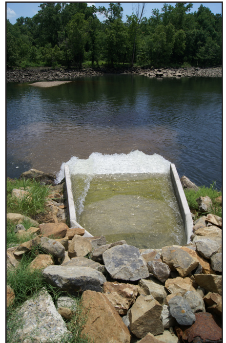
Water gushes from the low flow pipe system into the stream below the Tenkiller Dam. The low flow pipe system transports water from the surge tank at the hydropower plant to the stream.
