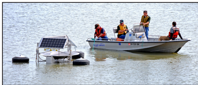
Placing the solar powered water circulators at Canton during the summer of 2014.
