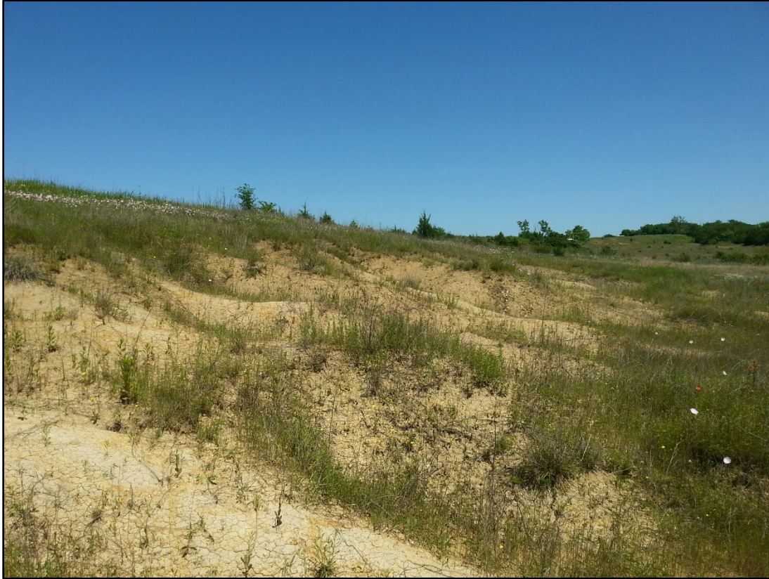
Figure 3.11-1. Erosion Rills on the Southern Edge of the City of Bonham Landfill
